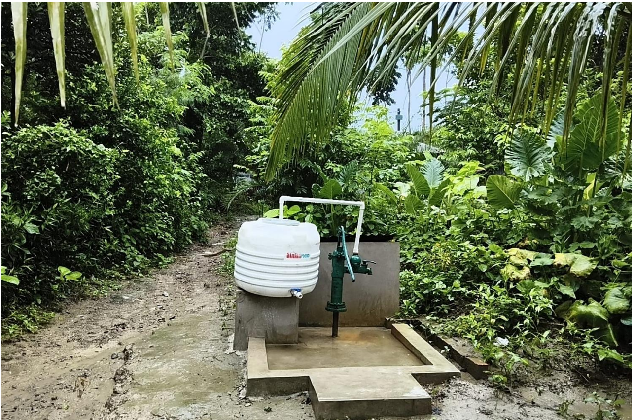
A bio-sand well installed under Project Well
